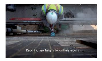
A £2,000,000 programme of remedial works has been underway on the power station since July 2007. The objective is to create safe access and slow down deterioration of the building through extensive roof, drainage and brick repairs. Works are being carried out by a restoration contractor in close liaison with English Heritage.
